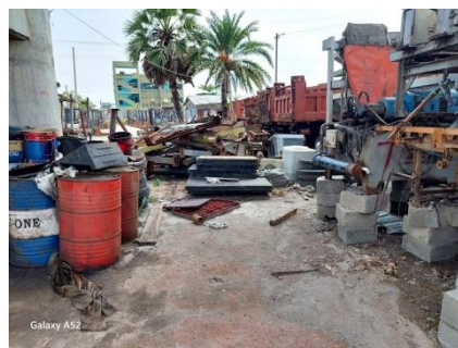
Figure 13: Daratana yard needs to be demolished (P-35/3)
