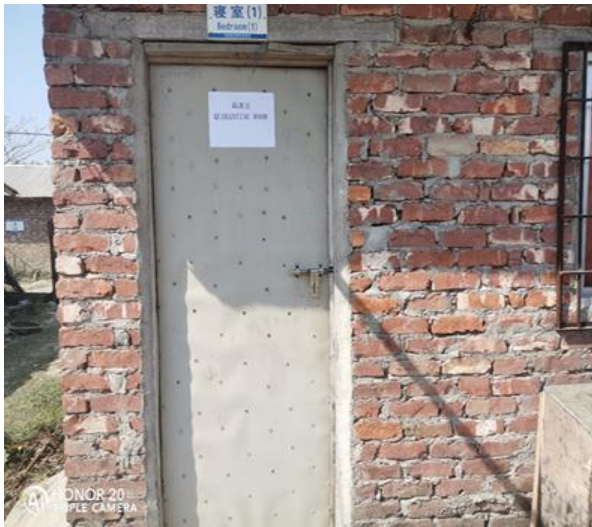
Figure 46: Quarantine room of Polder 43/2C
