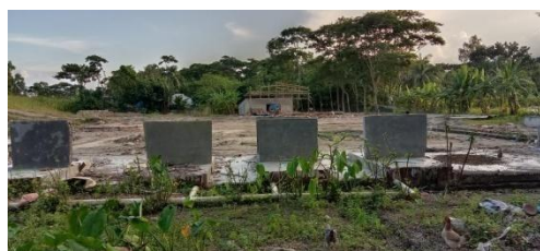
Figure 31: Demobilization has started in P-41/1
