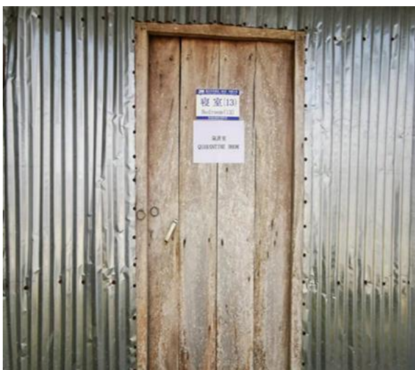
Figure 44: Quarantine room of Polder 40/2
