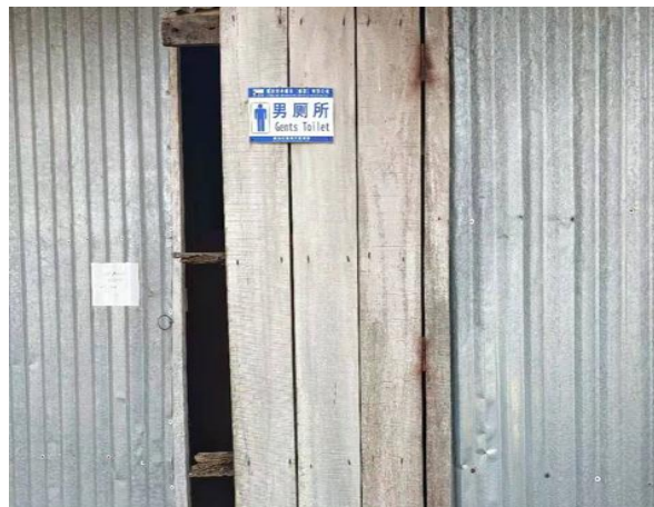
Figure 48: Toilet facility of Quarantine room of Polder 48
