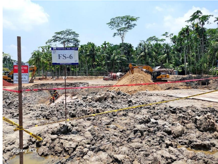
Figure 39: Demarcation in work site of Polder 39/2C
