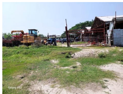
Figure 12: Remaining part of Tafalbari yard needs to be demolished (P-35/1)
