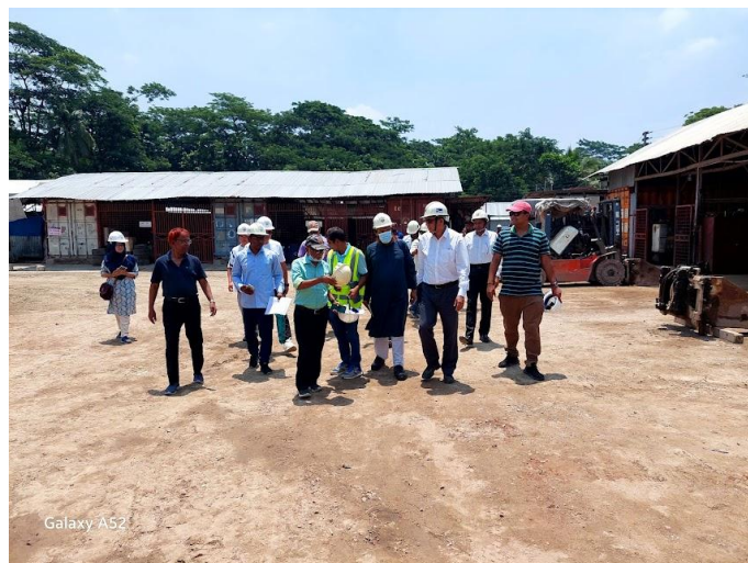
Figure 50: Senior Environmental Specialist of the WB monitoring construction activity in P-39/2C
