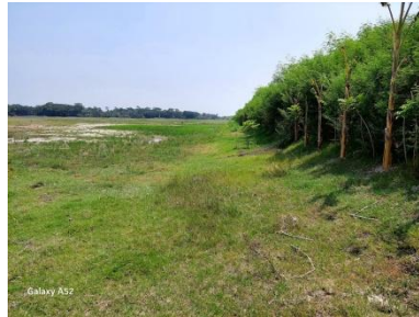
Figure 10: Demolished CC block yard of P-35/1 is being used for agriculture
