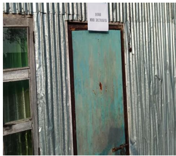
Figure 45: Quarantine room of Polder 41/1
